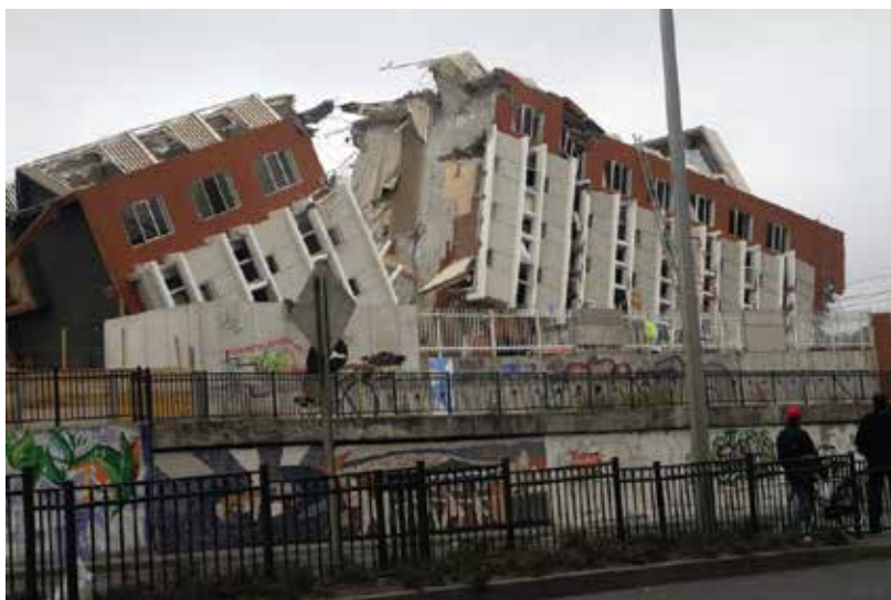
Fig. 9.09 : A damaged building due to earthquake
